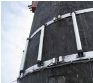
Array When the light tubes are mounted in arrays on the surface of the AtoN structure the light creates a good visual impression of the illuminated area. This allows the mariners to easily detect the structure.
