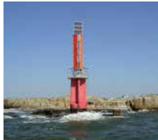
Leading lights Light tubes can be used to enhance the visibility of a leading line. Mounted vertically on the daytime panels, the leading light becomes very conspicuous in built-up areas with a lot of background light.
